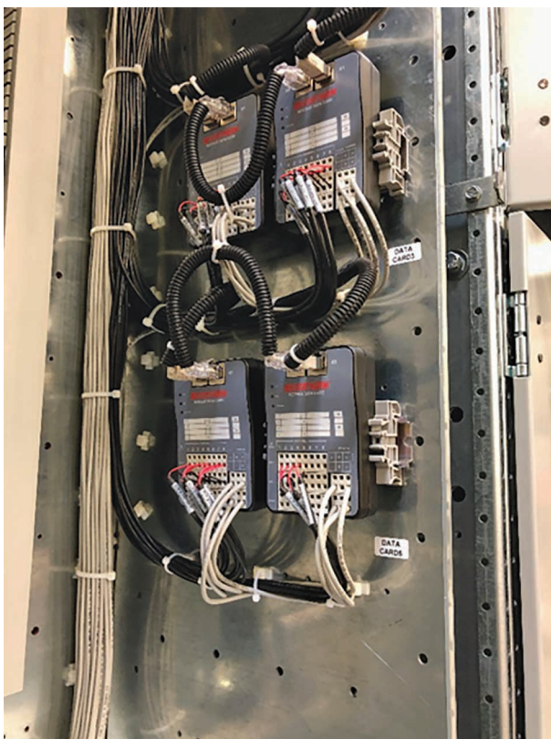
FIGURE 11. A collection of data cards for collecting and transferring temperature data to a host system for trending analyses.
